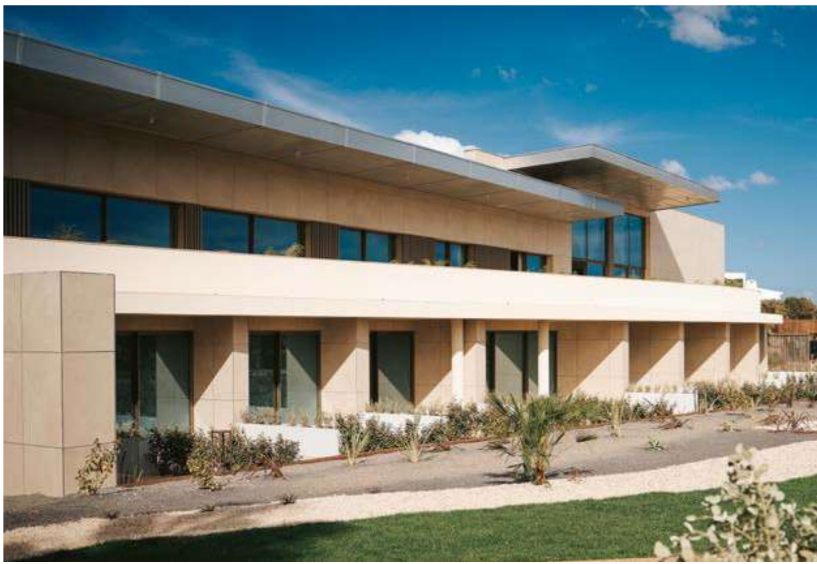
LIMESTONE SAND HOTEL LEGACY ITHOS _ PORTO SANTO, MADEIRA, PORTUGAL LEGACY ITHOS HOTEL _ PORTO SANTO, MADEIRA, PORTUGAL
